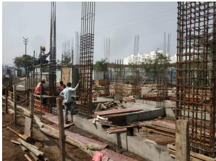
The casting of Plinth beams is complete and the casting of cols and first floor slab will be complete by end of this month.
