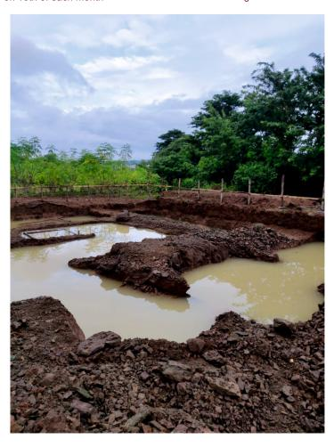
All the excavation done for footing was filled with water for 15 days as it was raining consistently.
